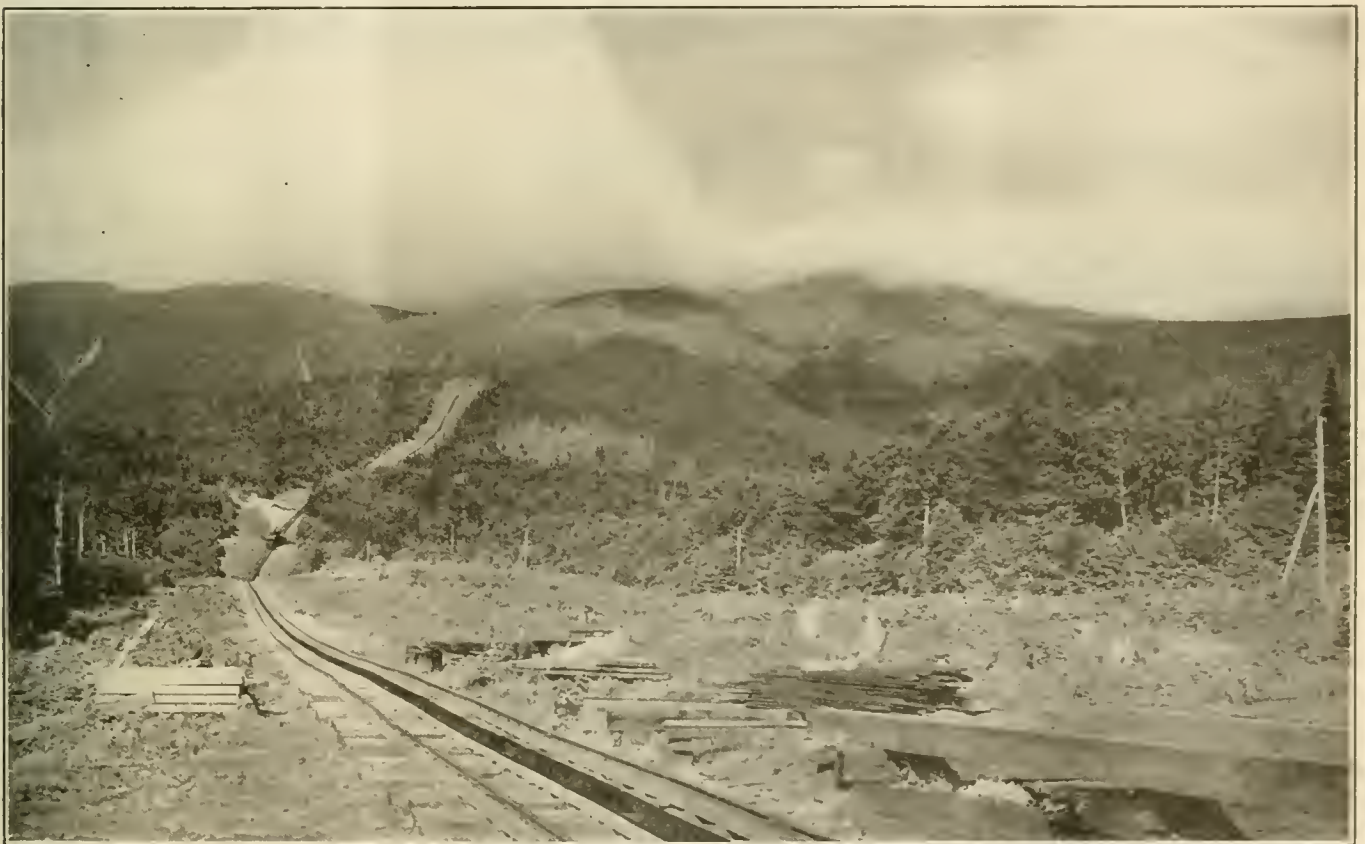
MOUNT WASHINGTON RAILWAY FROM THE BASE STATION.
